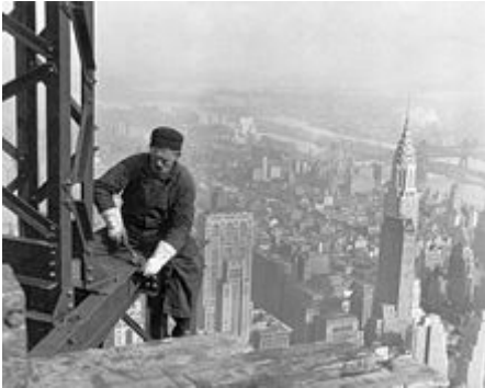
←A worker bolts beams during construction; the Chrysler Building can be seen in the background.
